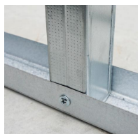
Vis ossature plaque de plâtre - montant + rail
