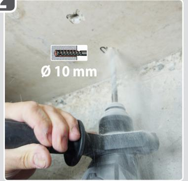
Percer  $\varnothing$  10 mm.
