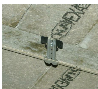
Suspente hourdis béton + suspente bois
